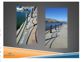
bollards are deteriorating to the point that they are not functioning how they are supposed to be functioning so depending on funding, it is likely that staff will be coming back with an annual program and one day have them all replaced.
